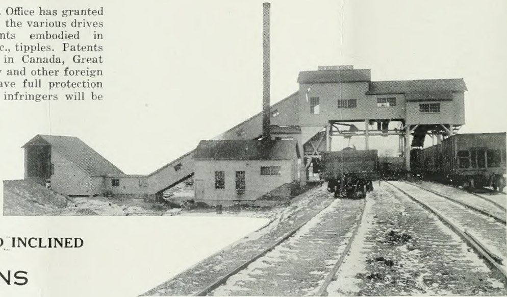
Complete Tipple and Power Plant using Jacobsen Balanced Horizontal Picking Table Screen—Typical Installation for a Stripping Operation
